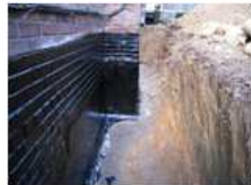
Exterior Foundation Waterproofing.
